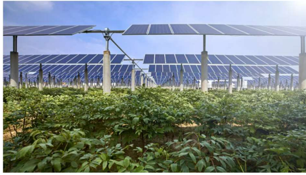
Offenes Agri-PV System 15
